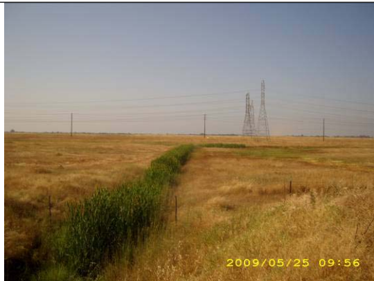
Westpark Outfall Channel at the Federico Tributary.
