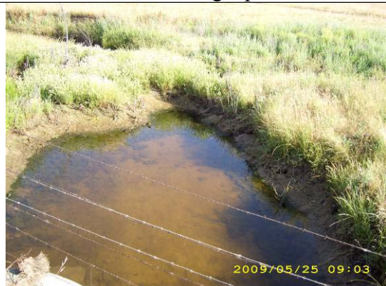
Curry Creek Main Branch, at Culvert Plunge Pool,
