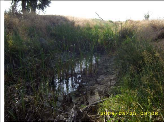
Curry Creek Main Branch – Example of a Dry Season wet stretch of channel. Also demonstrates the up and down nature of the channel invert.
